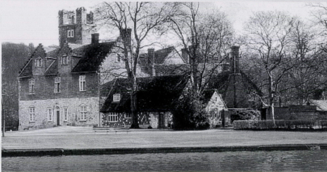
Rear view of the Abbey Photos: Bisham Abbey National Sports Centre
