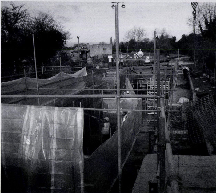
Work in progress at Godstow lock
