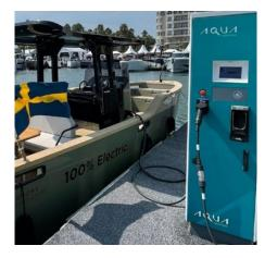
first major European inland lake installation. The electric boat fast chargers have AC and DC 25kW-150kW power and can be used for everything from recreational electric and hybrid boats to electric jet-skis, super yacht tenders, commercial vessels and passenger ferries. Aqua will own, operate, and maintain the network with their own cloudbased system and users have an app with maps of charger options and navigational aids to charger locations.
